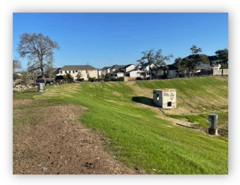
13. Wrap the inlet riser screen assembly with silt fence if loose and disturbed soils still exist in the pond site. Leave wrapped until well vegetated, then remove.
