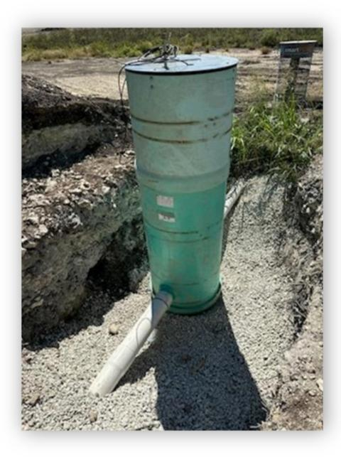
7. Connect the pipe from the inlet riser screen to the INLET side of the vault. The vault should be labeled for inlet and outlet side, but for reference, look through the trap door in the vault lid to confirm the location of the inner valve assembly. The valve assembly will be bolted through the vault wall on the inlet side of the vault. The valve discharges into the vault chamber when opened.
