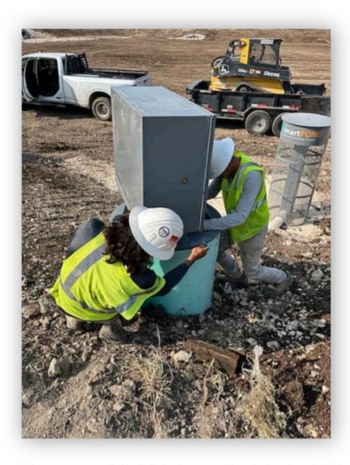
10. Once the vault and inlet screen are installed and all plumbing is complete, final earth work and backfilling may take place.
