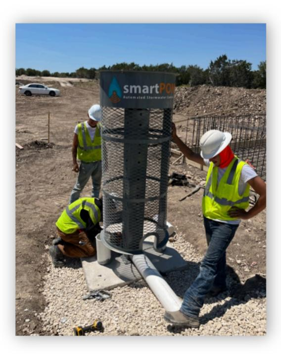
6. Attach the discharge pipe to the inlet screen riser and route to location of the valve assembly
