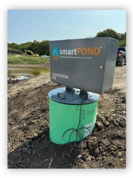
11. With final earth work completed, activation of the vault valve may be requested. A manufacturer-certified technician will arrive with the solar kit, battery, and control electronics to activate the system and certify for warranty.
