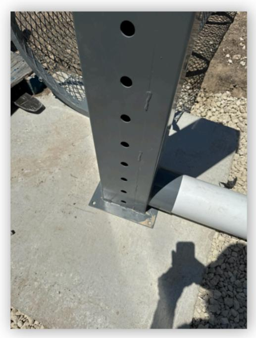
• Slide the outer screen around the perforated square tubing and secure to the pad using 3/8" concrete anchors.
