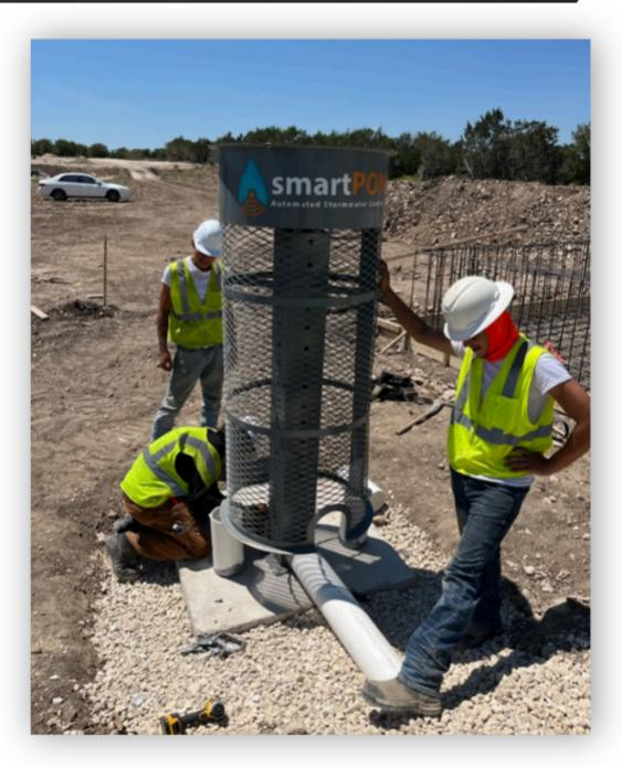
• Attach the discharge pipe to the inlet screen riser and route to location of the valve assembly
