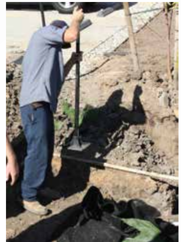
Figure 19: Compaction of side is critical in order to keep soils from settling around the tank.
