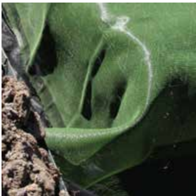
Figure 17: fold corners flat against the tank
