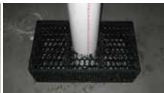
Figure 13: Place inspection port into underdrain module
