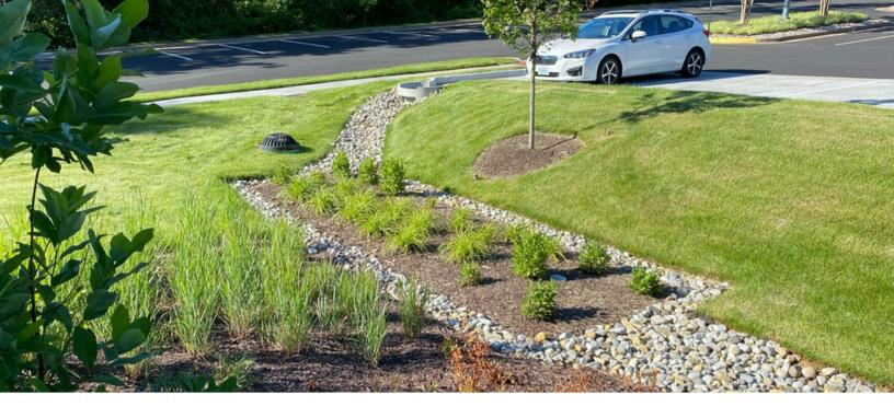
FocalPoint's advanced design sets it apart from traditional bioretention systems. With an infiltration rate of 100 inches per hour, far exceeding typical bioretention soil mixes, it rapidly processes runoff, minimizing required footprint while maintaining peak performance with minimal maintenance. Its modular nature allows seamless integration with other Low Impact Development (LID) strategies, such as bioswales and stormwater planters, making it ideal for both urban and rural applications.
