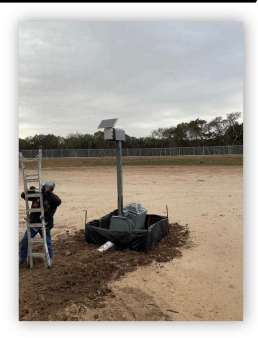
9. A manufacturer-certified technician may now be requested for activation of the device. The technician will furnish the electronics kit, battery, and solar panel to complete activation of the rotary weir and certify for warranty.
