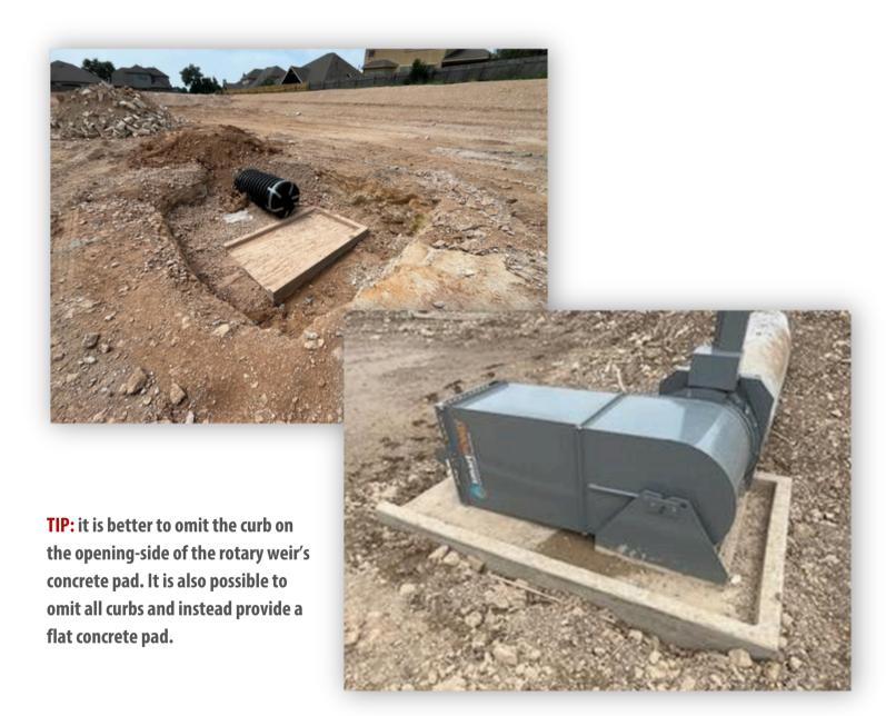
4. Using an excavator or other heavy equipment, carry the rotary weir into position and attach to the drainage pipe (connection details vary based on specified drainage pipe type)
