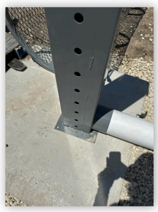
5. Slide the outer screen around the perforated square tubing and secure to the pad using 3/8" concrete anchors.
