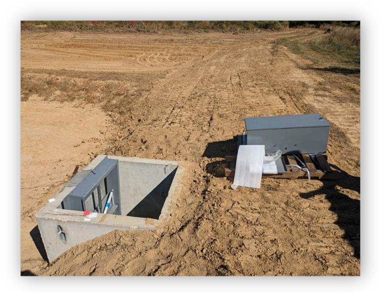
4. Align the slide gate's orifice with the knockout of the concrete manhole and use a hammer drill to set 3/8" anchors through the slide gate's frame. At least 3 anchors per side, and two in the bottom are required to secure the gate.
