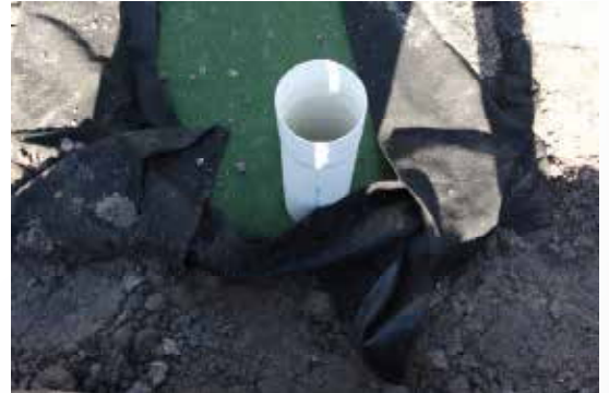
Figure 16 (Below): Cut an "X" into Biaxial Mesh to accommodate pipe penetration
