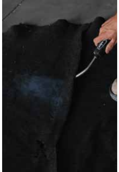
Figure 29: Geotextile being melted together with a torch.
